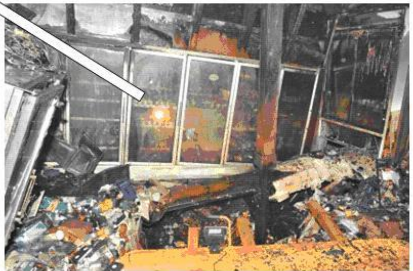
Delicatessen view of rear wall coolers. Note framing above that rose to ceiling, creating a dividing wall between the store and a rear apartment.
