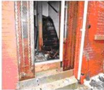
Main entry to basement staircase on Side #2 Door 2B
