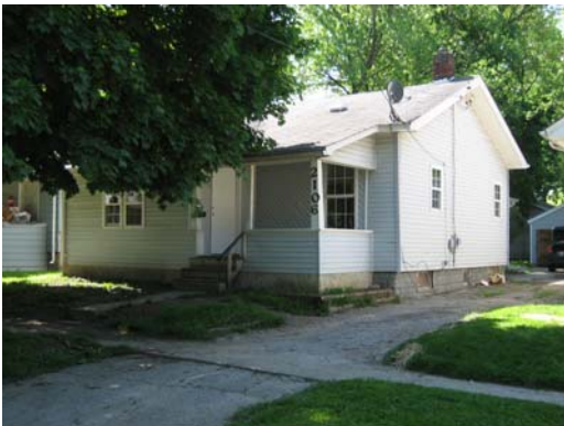
A vacant house at 2106 Dakota undergoing renovations. Fire occurred here on August 16, 2006. No firefighters were injured.
