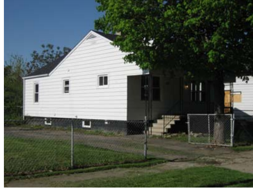
A vacant house undergoing renovations at 939 Pettibone. Fire occurred here on October 31, 2006. No firefighters were injured.
