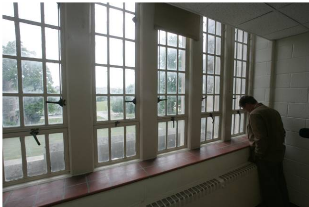
Figure 11. Typical Set of Windows in Norris Hall
