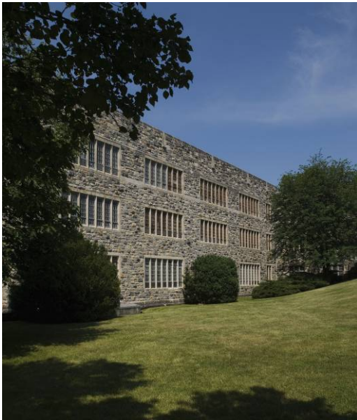
Figure 10. Norris Hall Classroom Windows, Grassy Side
